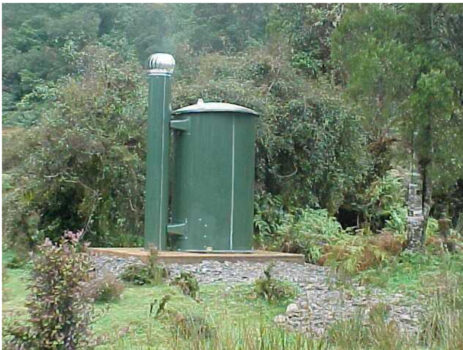
Figure A2: Single Vault Toilet New Zealand
