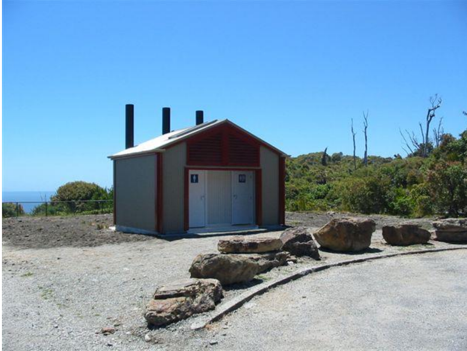
Figure A3: Multiple Vault Toilet New Zealand
