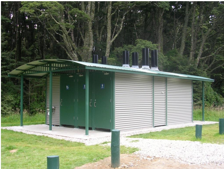
Figure A4: Multiple Vault Toilet New Zealand
