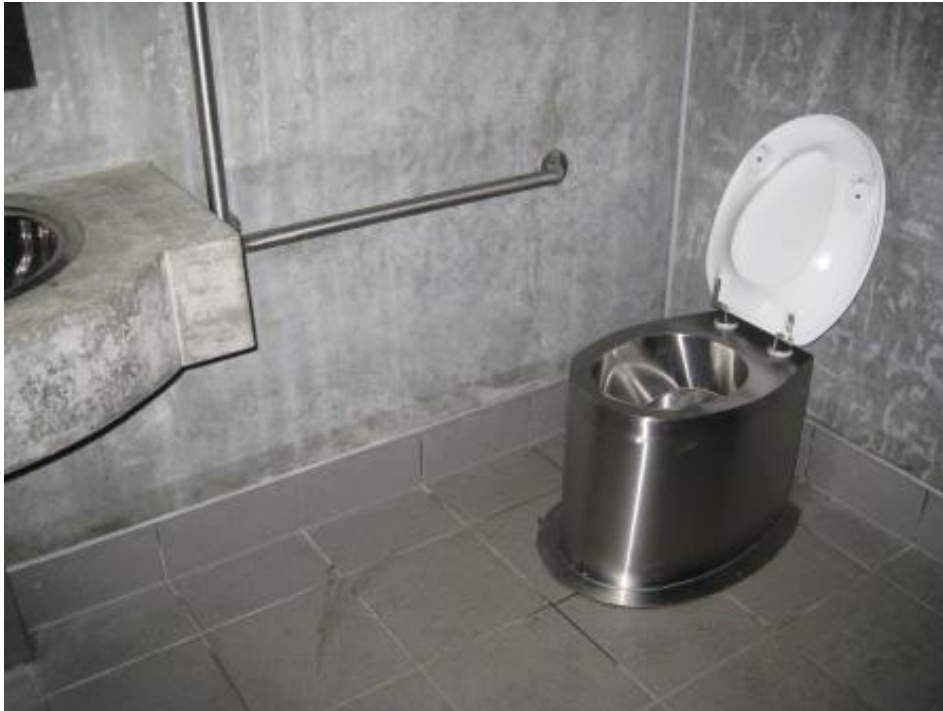
Figure A1: Vault Toilet Interior New Zealand
