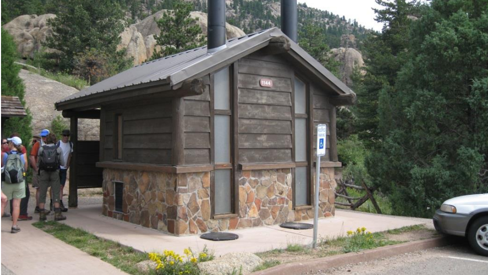
Figure A5: Vault Toilet USA
